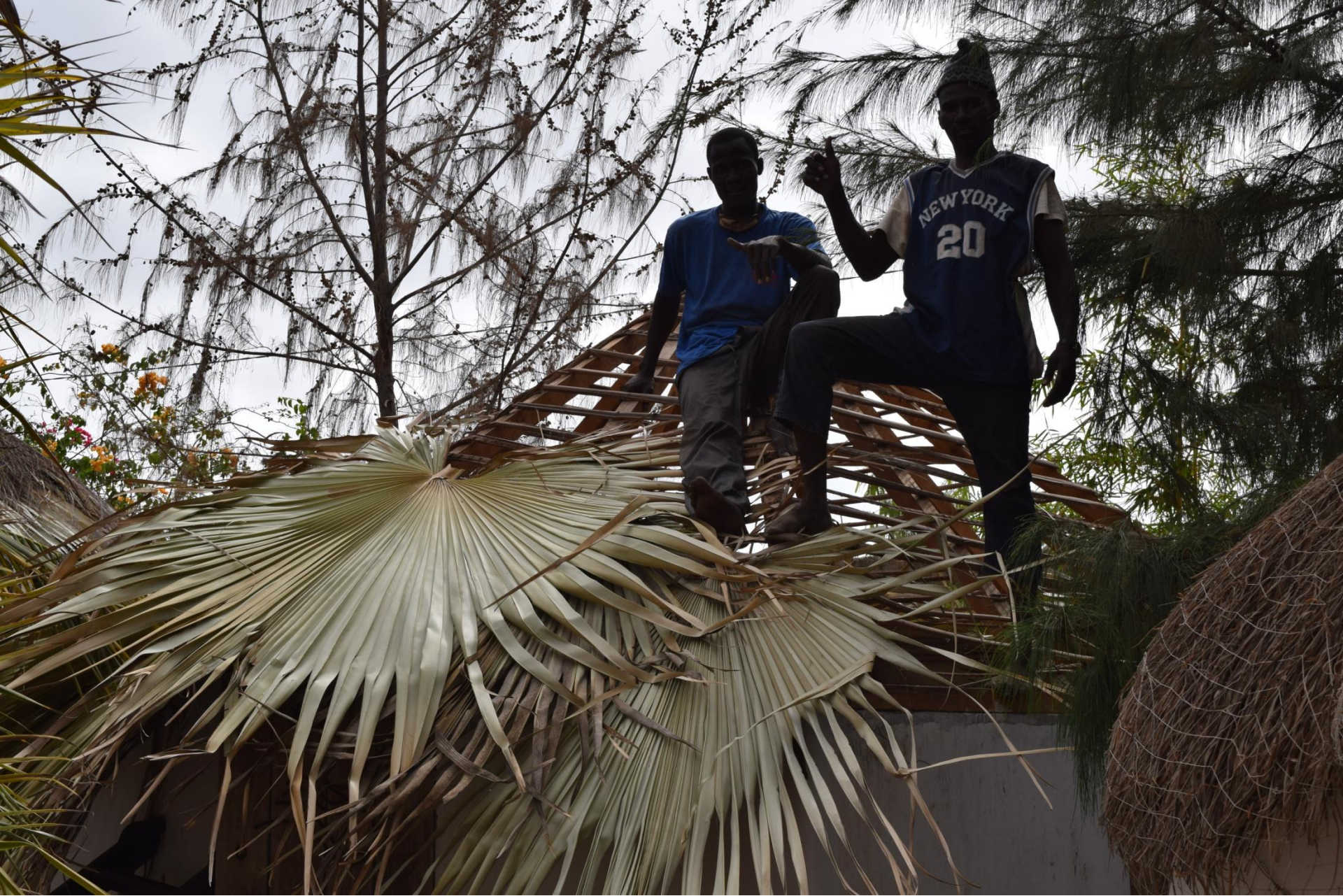
Putting a new roof on the hut
