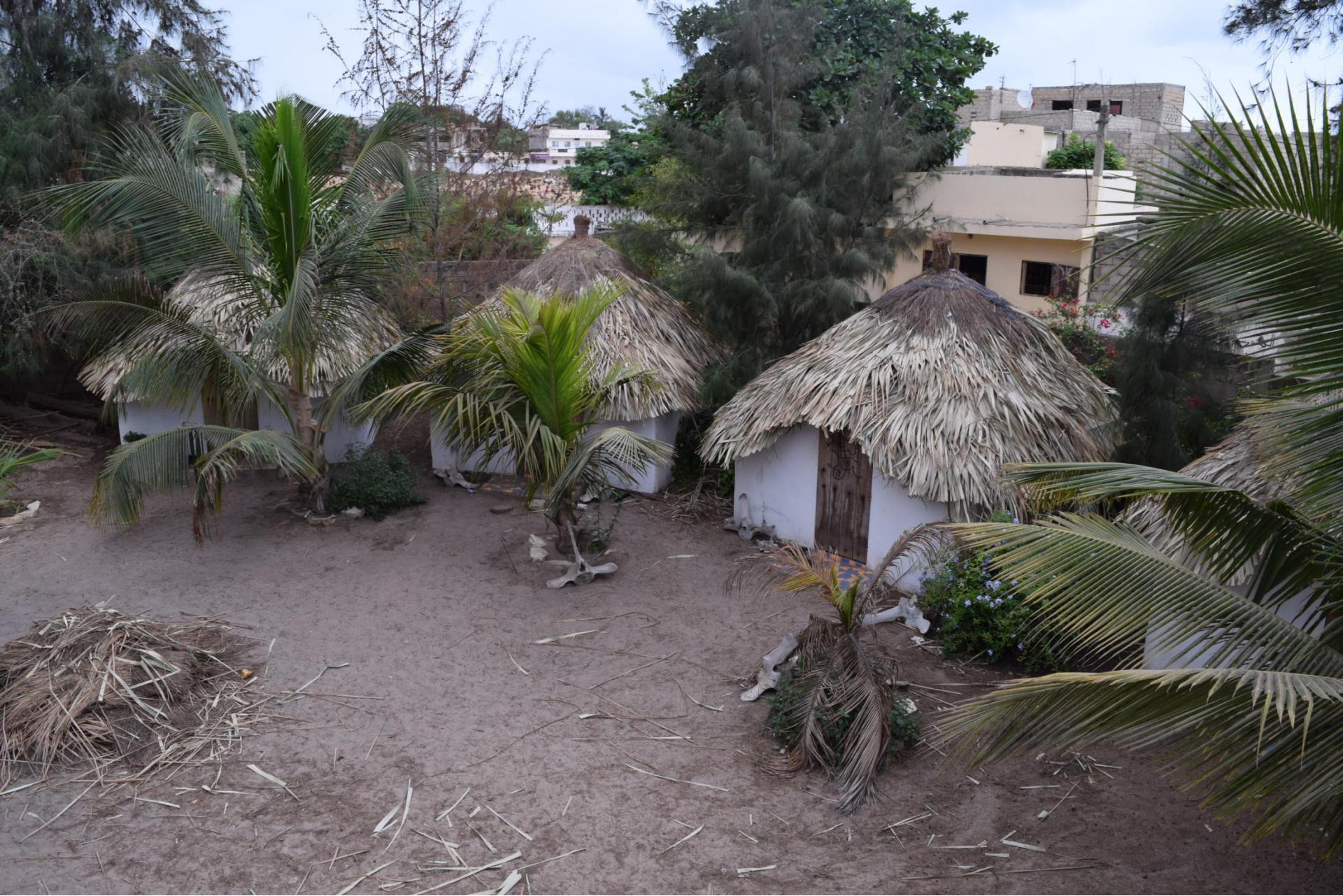
Finished new roofs on the huts
