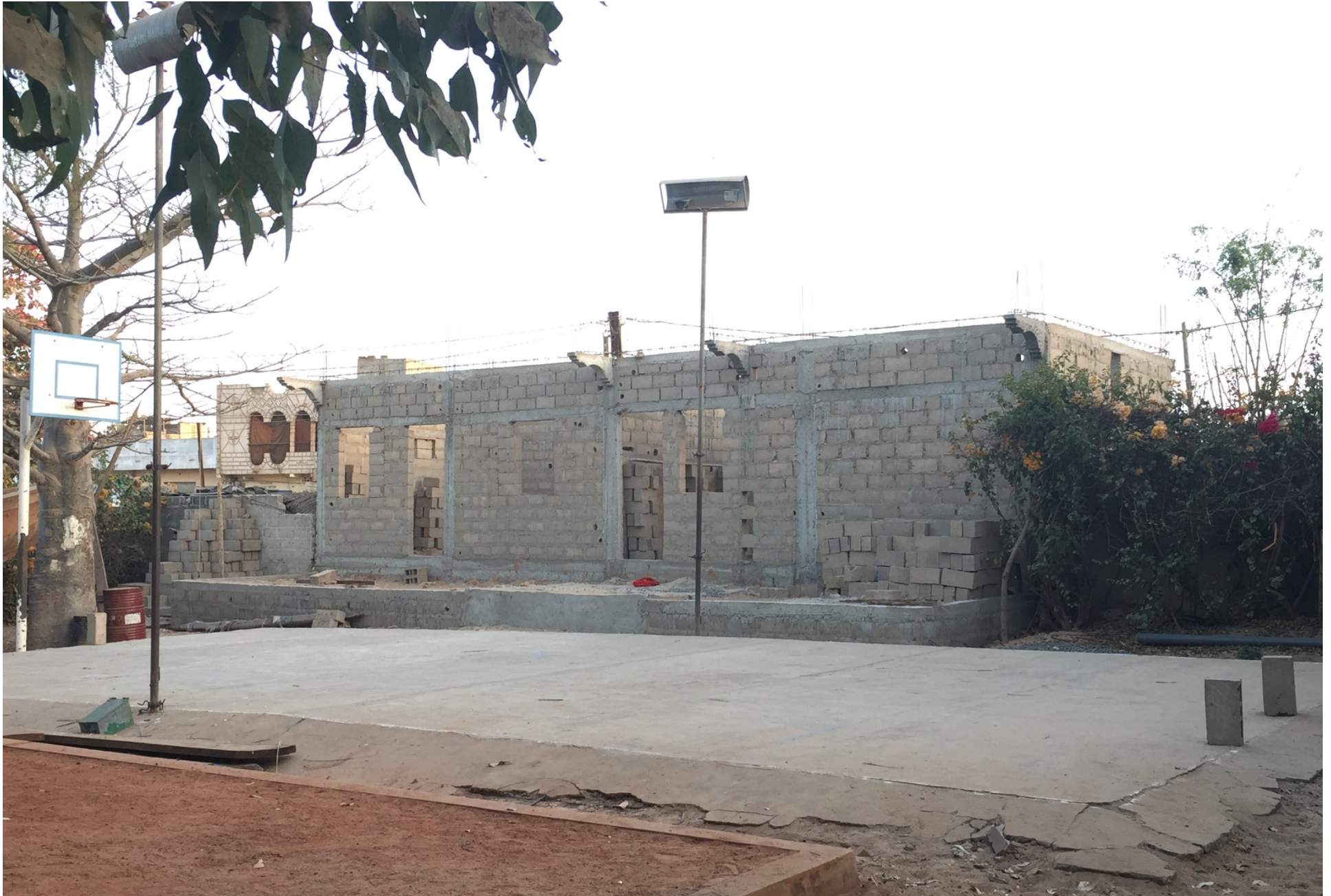
Recording studio under construction
